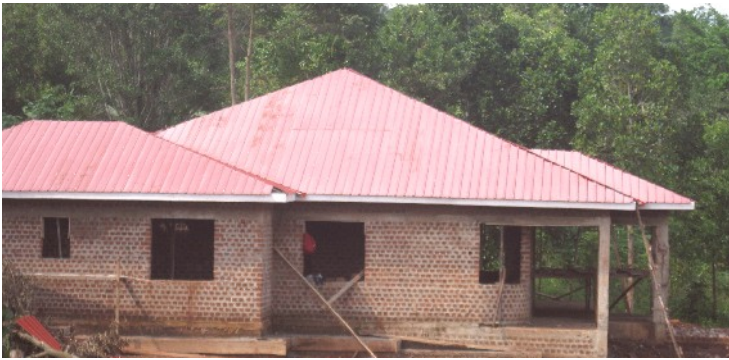
The roof goes on the missionary house!
